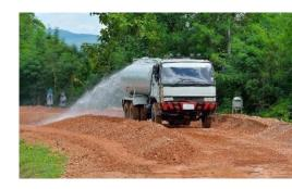
1. Grade the road according to the road design specifications desired, placing graded material to the side in a windrow.
